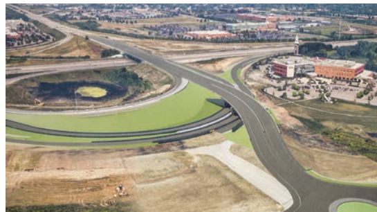
Using InfraWorks, EMH&T was able to measure bridge clearances far quicker than in other programs.
