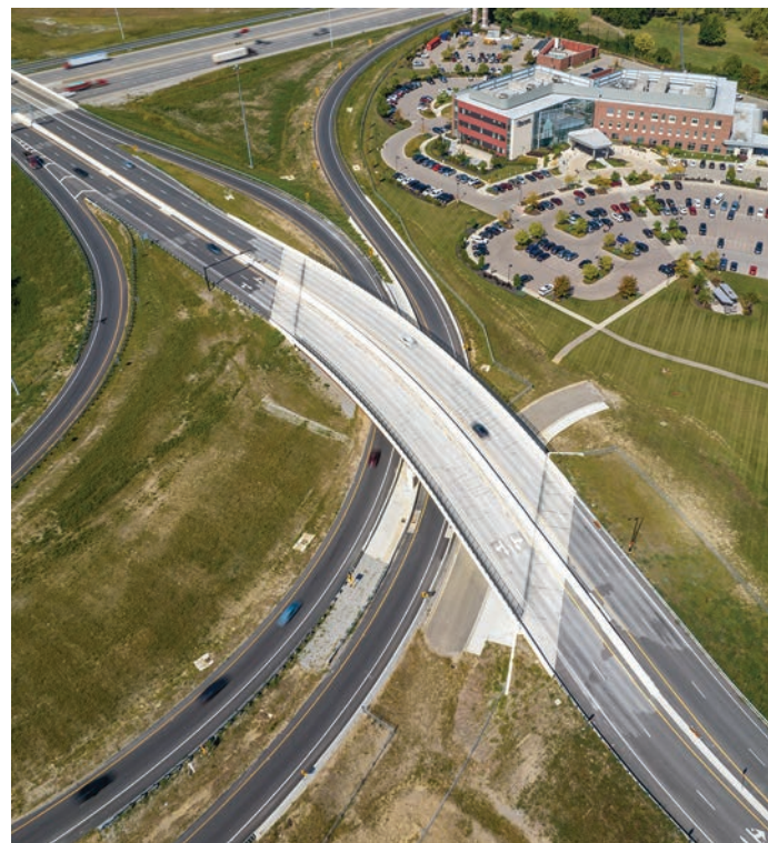
SR 129 and I-75 interchange redesign included a new bridge over re-aligned I-75 ramps.
