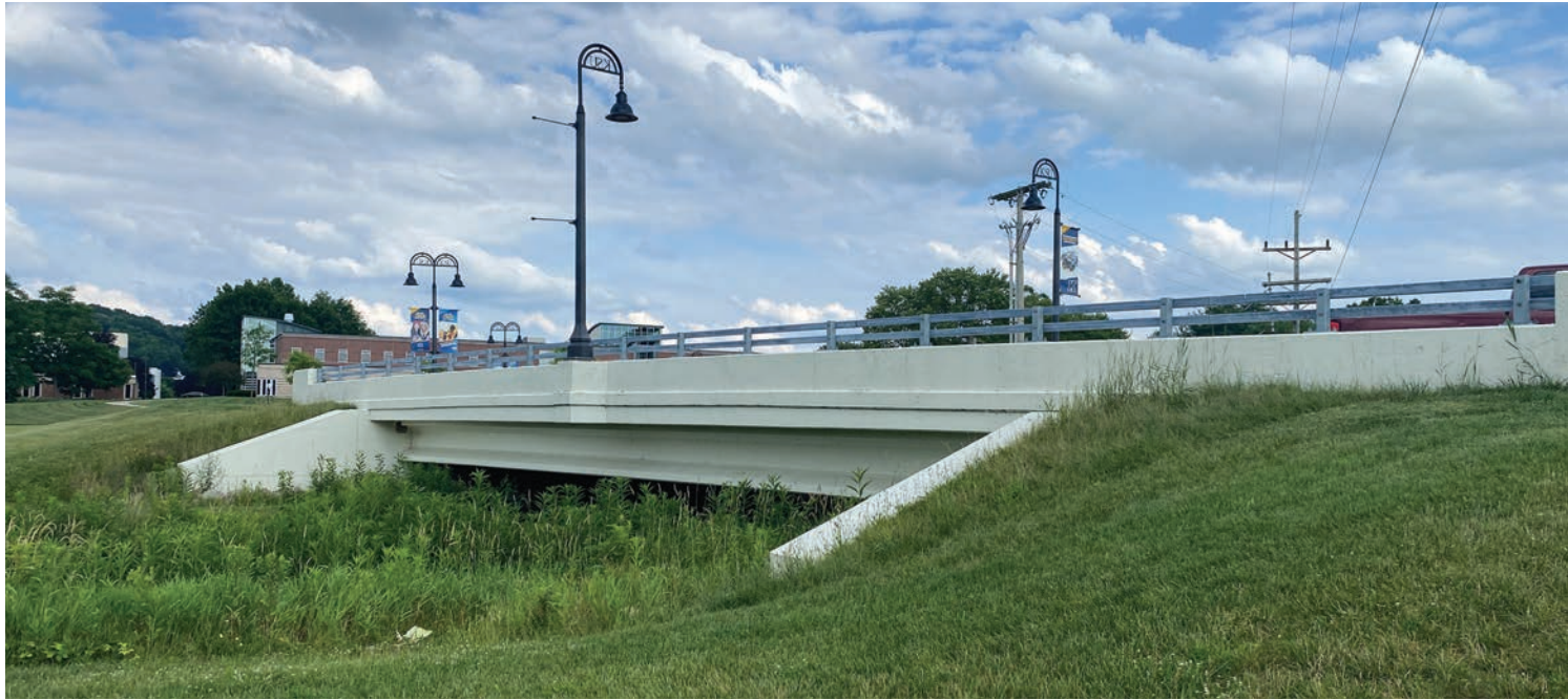
Kent State University Tuscarawas Campus new entry bridge
