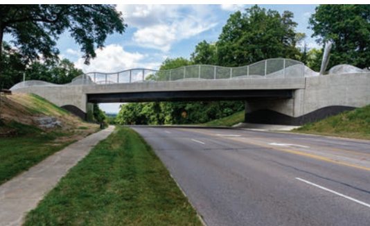
Ridgeway Road Bridge over West Dorothy Lane in Kettering, Ohio
