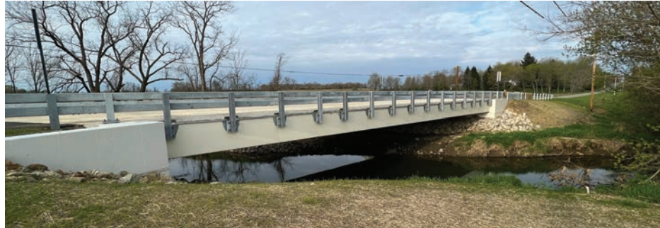
Lock Road Bridge in Knox County, Ohio
